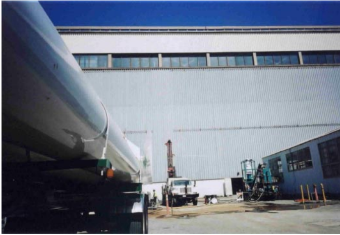
Nitrogen tube trailer, drill rig and injection trailer
