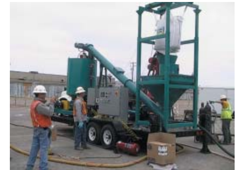
New large-scale material mixing and injection plant in use.
